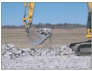
Excavator removing broken jointed reinforced concrete
