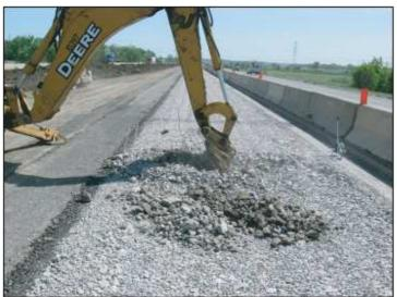
Jointed reinforced concrete pavement
