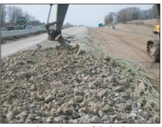
Excavator raking rebar out of the broken concrete
